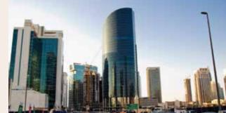
KCPC designed and built this prestigious commercial tower consisting of 3 basements, ground floor and 36 floors (30 floors of office space, two levels allocated for retail establishments and 6 parking levels). The tower boasts a grand main entrance with a 12 meter high atrium containing a specially- designed curtain glass wall.
